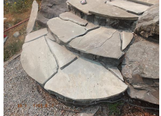
Old stone removed, new stone cut
